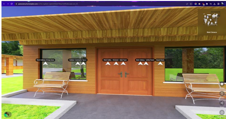
Figure 6: Main entrance of the building
