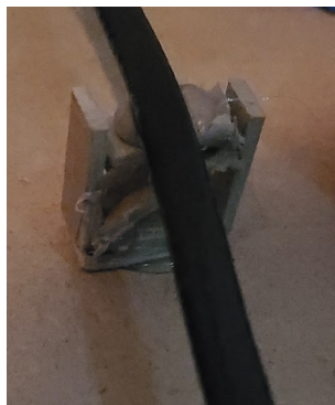
Figure 11: Standoff holding up the de-icing wire
