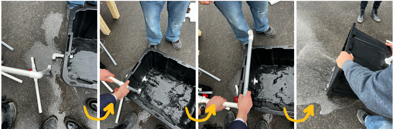
Figure 11: Step-by-step images for freeing the hydroponics reservoir.
