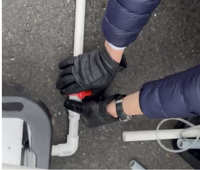
Figure 9: Ideal grip when operating the stopcock on the drainage pipe.
