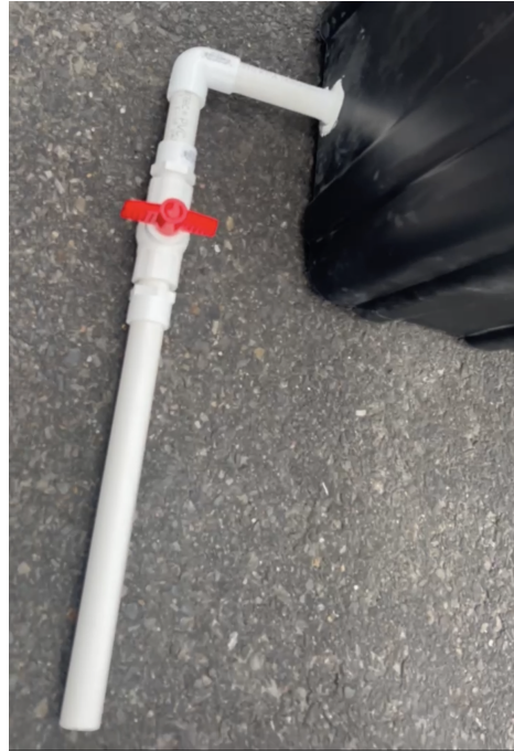
Figure 4: Final assembly of drainage pipe.
