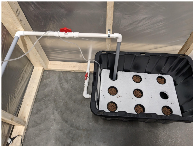
Figure 5: View of the drainage pipe inside the greenhouse.
