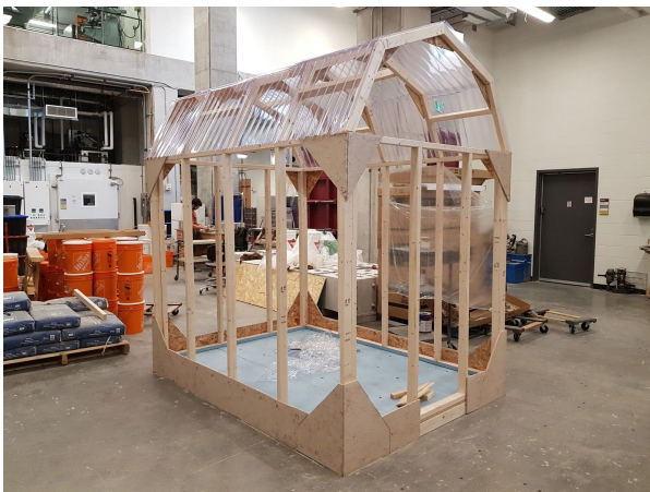
Figure 2: Documentations (images) of the current construction of Prototype 3 (more in appendix)
