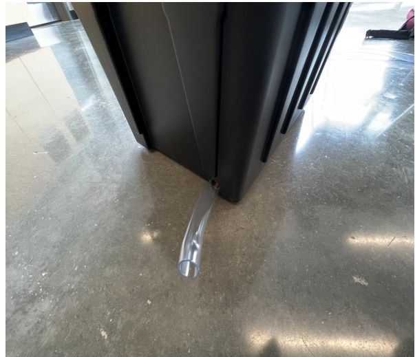
Figure 6: Inner pipe exit
