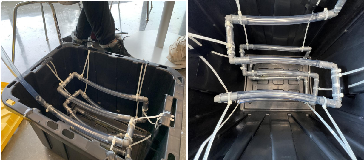
Figure 3: Inner pipes inside chamber box
